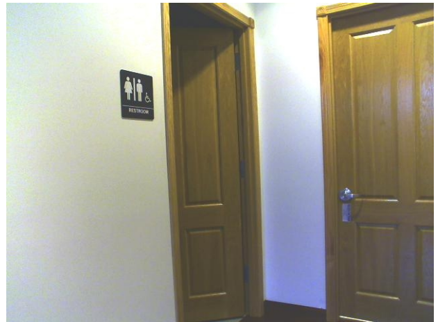
Restroom , Wall Signage : Wall Signage Height
