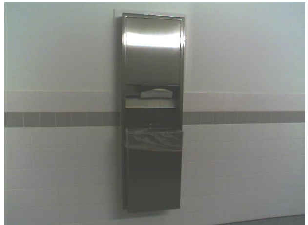
Restroom , Dispensers : Dispenser Height
