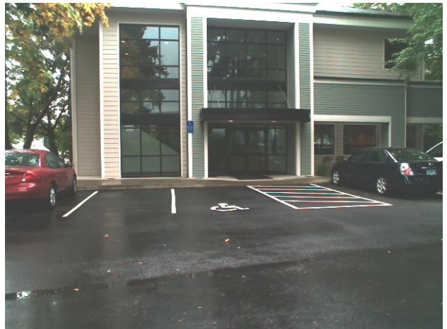
Parking Lot : Less Than Minimum Required Parking Spaces
