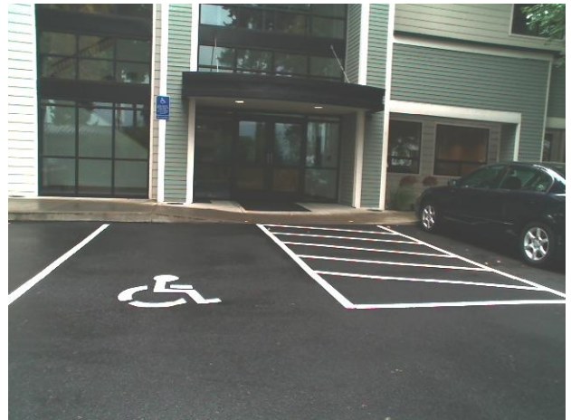
Parking Lot , Parking Space : Access Aisle Slope
