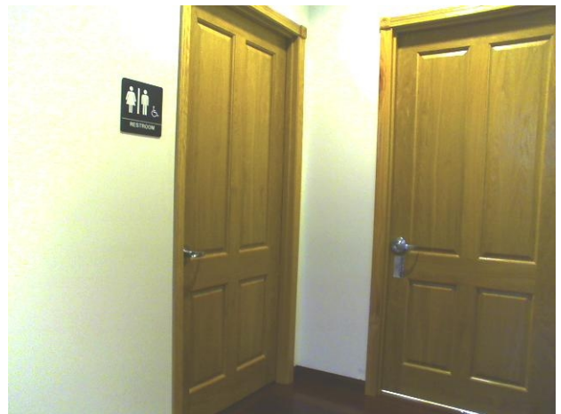
Restroom : No Visual Alarms
